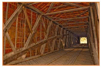
Theodore Burr first used this arch design for a bridge constructed over the Hudson river in 1804. The arch is bolted to the trusses and connects to the face of the abutments. The truss rests on the concrete abutments.
