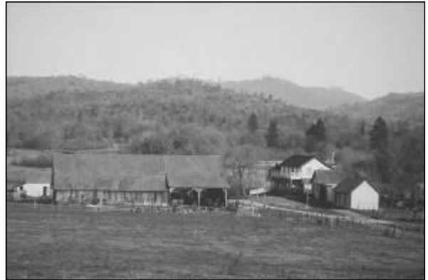
Barn and Anthony House
