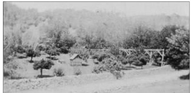
Flume to deliver Kentucky Creek water to field
